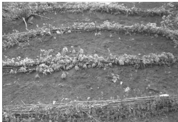
Fig. 1. Beech tree mattress after being set up (2004), in the former bauxite quarry of Zece Hotare, Bihor
